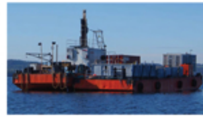
Fig. 2. The drilling barge at southern Lake Vättern
